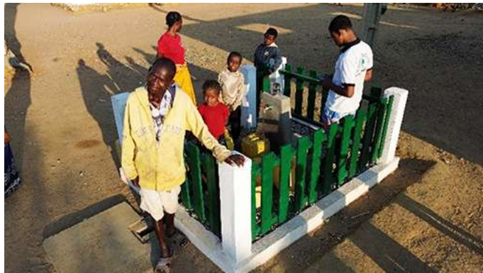
A village "water station" guarded with a fence, a concrete slab and a hand pump that is tamper-free to keep it from being stolen
