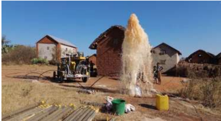
below: Water gushing from a newly-drilled well
