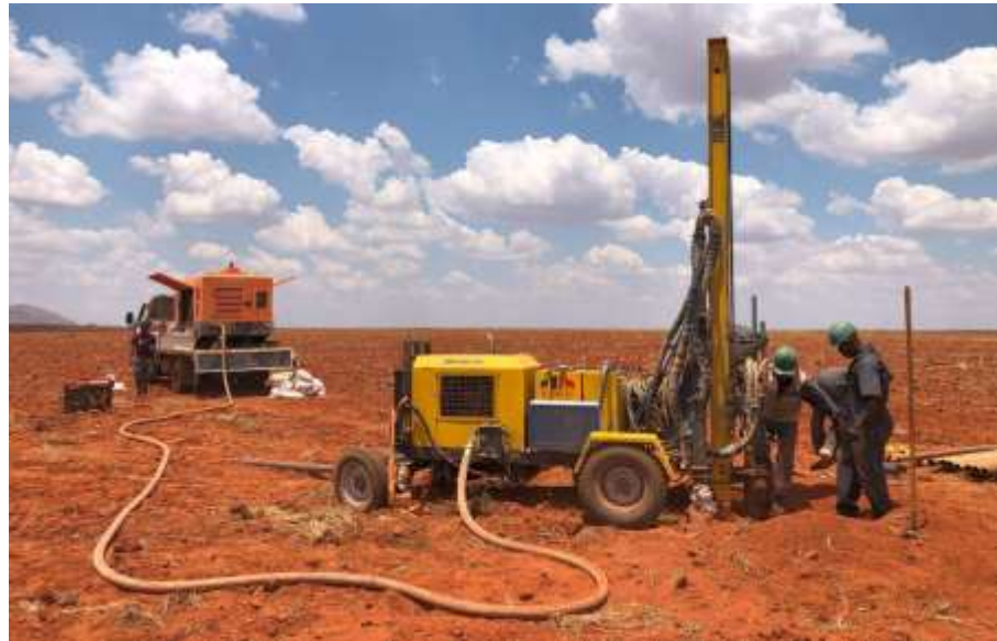
Drilling a new well
