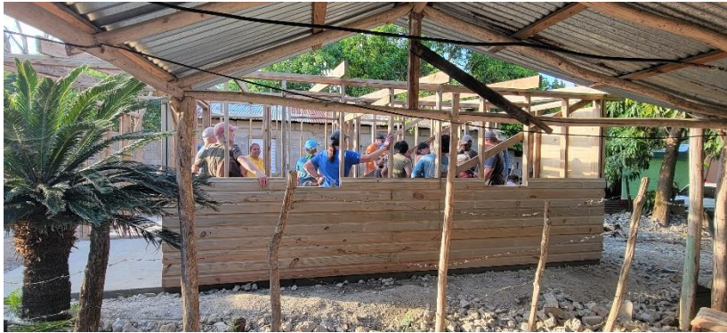
House project taking shape
