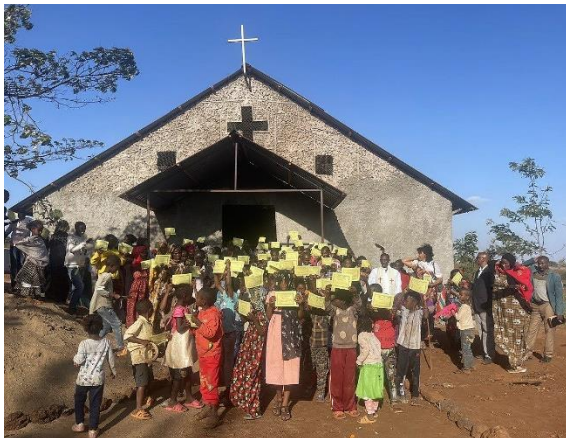
Dirib Gombo Church - some of the group baptized in December 2022. This church was rebuilt in a better way after 11 years, using metal, local rocks and chicken wire, since termites eat away the wood parts of buildings.
