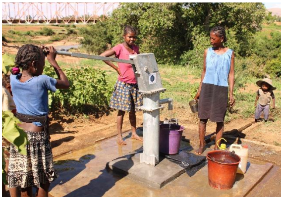
Repaired water well
