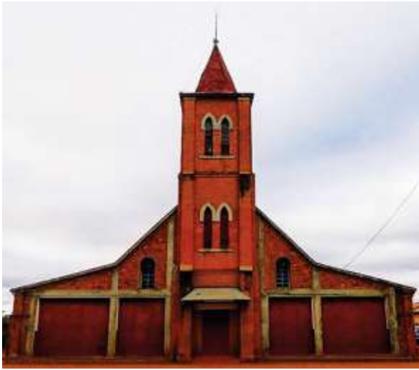
Some Toby buildings near Antsirabe were damaged by a rare Earthquake in 2020 - Friends of Madagascar Mission helped rebuild the buildings
