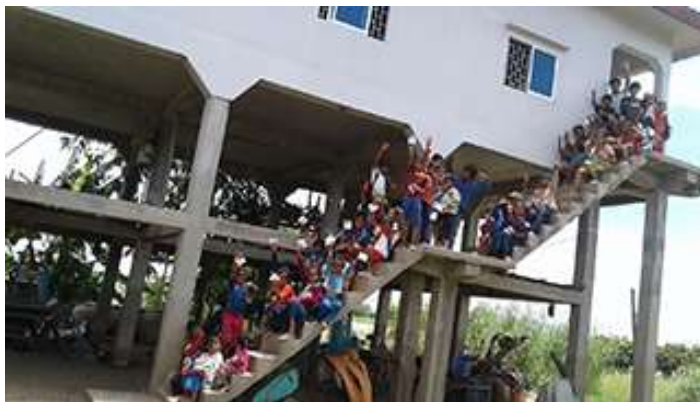
Stairway at LCMC Cambodia / ALWM Mission School In Preh Vihear, Cambodia
