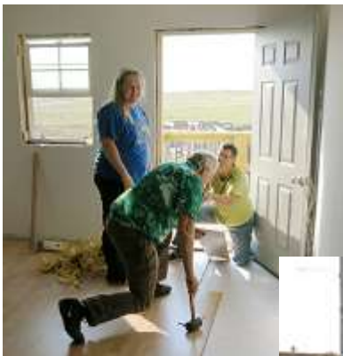
CTK members finishing a construction project at Oyate Concern Christian School
